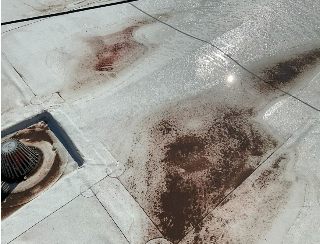
8. View of the ponding located next to the roof drains.
