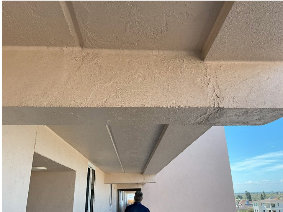
29. View of the previously patched beam outside of Unit 503.
