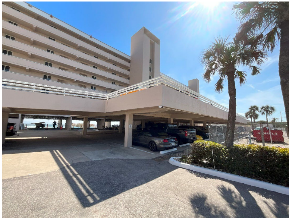
42. View of the Parking Deck.
