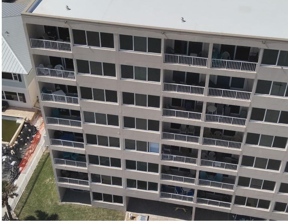
9. View of the northeast elevation.
