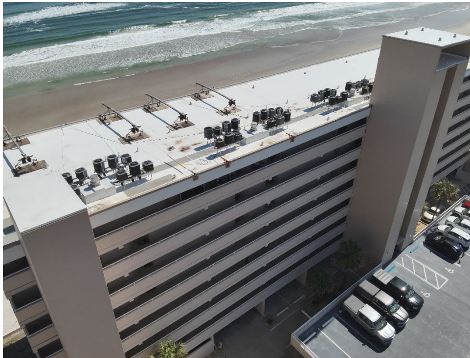
10. View of the southwest elevation.
