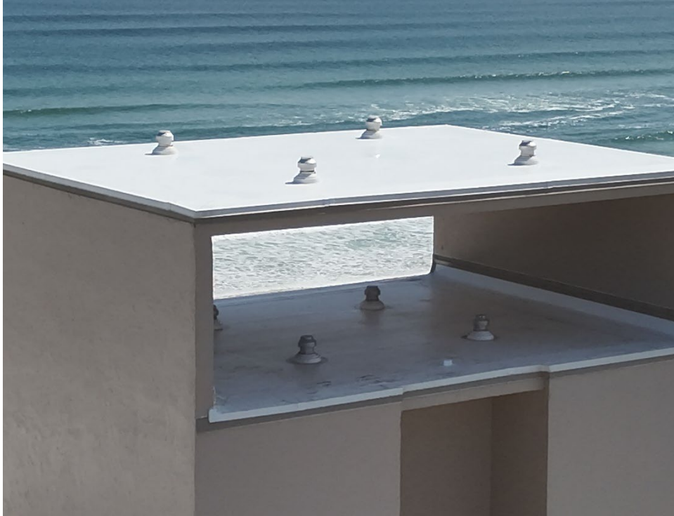
5. View of the flat roof membrane on the Elevator tower.
