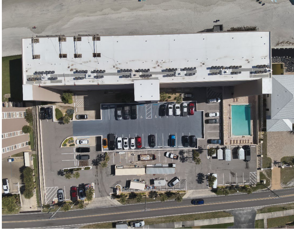
3. View of the roof of the subject complex.
