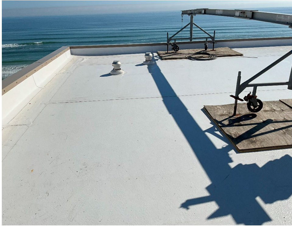
7. Additional photo of the flat roof membrane on parapets.
