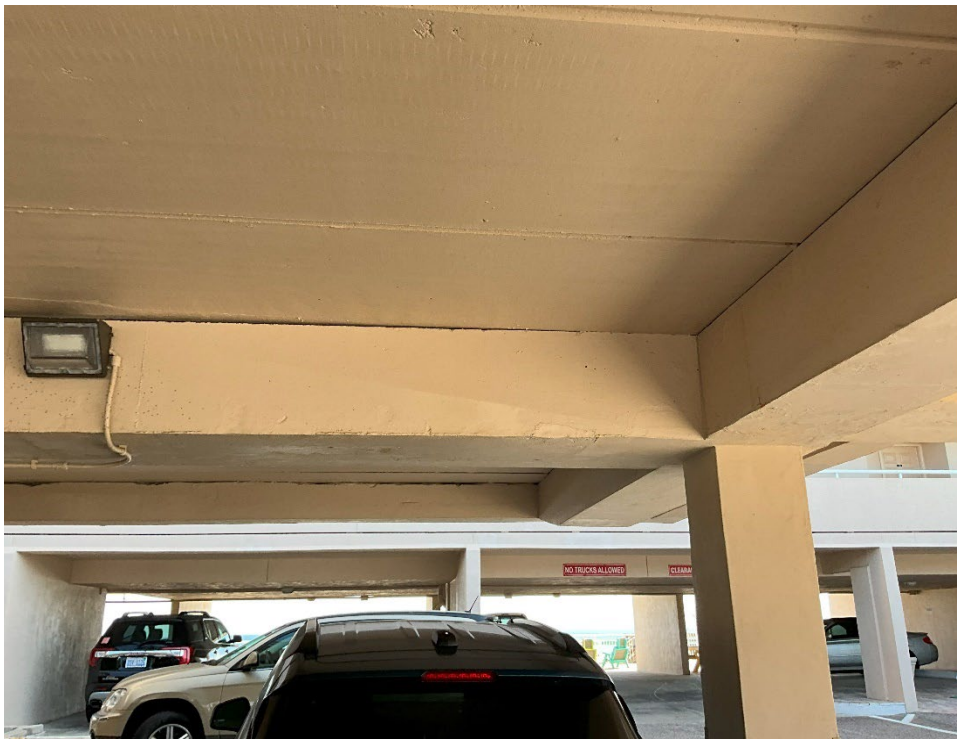
44. Typical beams and columns under the Parking Deck.
