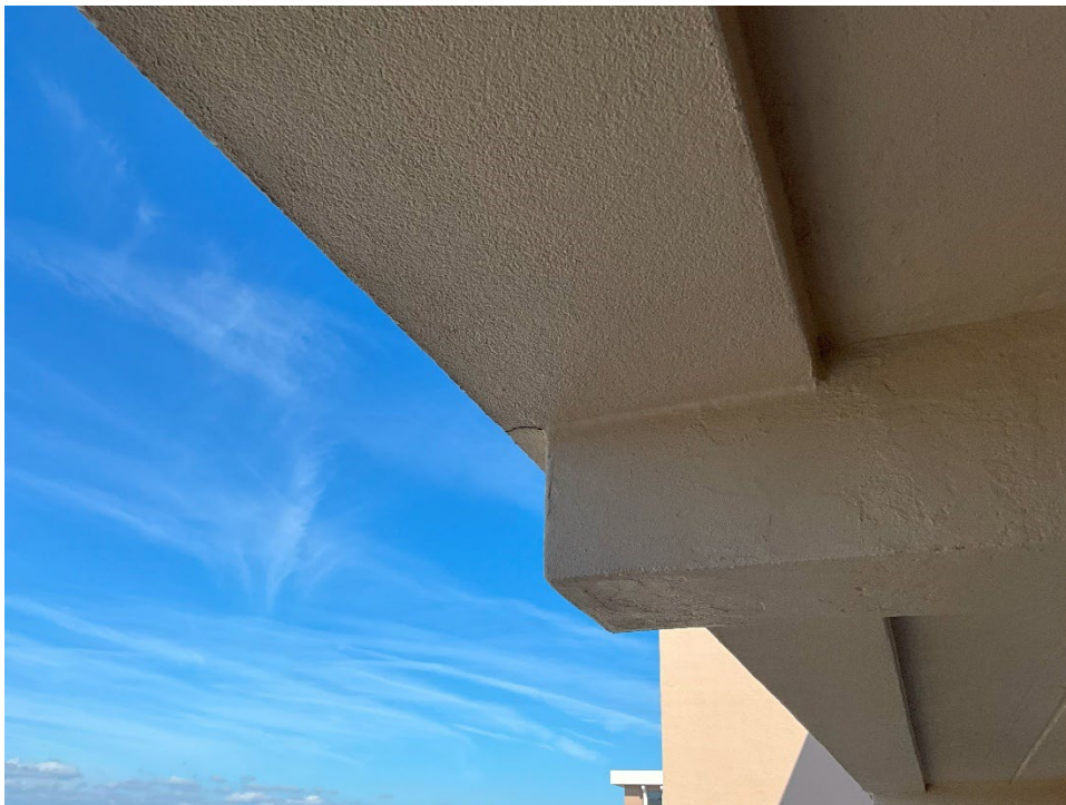
32. View of the crack in the underside of the Breezeway slab outside of Unit 509 and 410.
