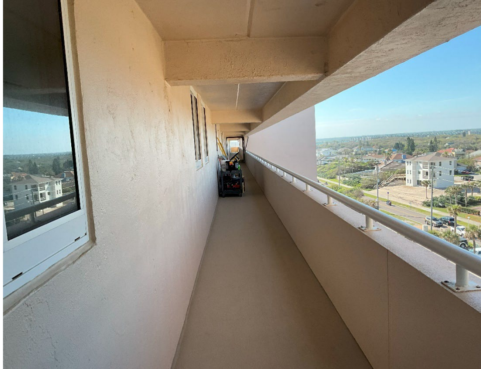
11. View of the 7 th floor Breezeway.
