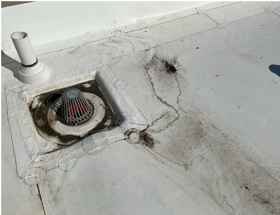
6. View of the roof drains located on the main roof.
